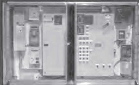
Pad Mounted Control Packages
