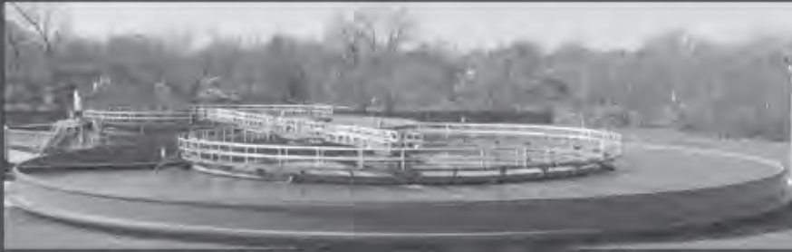
Wastewater Treatment Solutions
